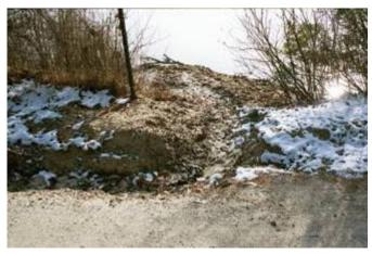
2. The brook/spring inlet on the northwest side of Halfway Pond is continually at risk. Road runoff flows into this area. The pipe under the shore road connecting the inlet to Halfway Pond is often partially crushed by large vehicles.
