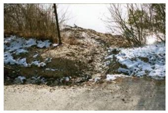
Recently, the Highway Department made at least six new cuts through this narrow buffer. There are no catchment basins along this section of road, and careful planning would be required to create ones which would not adversely affect this fragile area. In places, the cuts have eroded severely and carried a great deal of sand and silt into the pond.
